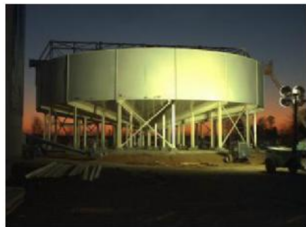
Lintech has just got an order to build two 45m dia elevated thickeners like in picture above for FLSMIDTH MINERAL, Australia for LIHIR Gold Mining – Papua Newguinea
