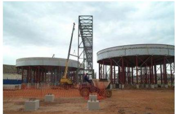
Site Shell erection thickener reference
