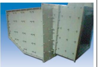
View of launder box wet application which the liner was bolted. The wear bar is installed at "dead bed" area and bottom surface.
