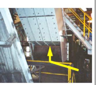
Back view of the chute into which the liner was bolted. The liner is situated at the main impact zone in the chute at the change o direction point
